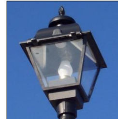
Photo C. The white globe visible to the eye in this post top fixture is decorative; the lamp is in the top of the fixture.
