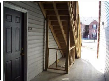
Photo D. Example of breezeway stairs where the stair risers are solid and don't allow light through into the breezeway. Also, an example of a solution to often unused space under stairs where people may hide.
