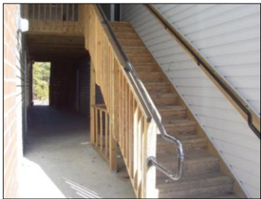
Photo D. Example of breezeway stairs where the stair risers are solid and don't allow light through into the breezeway. Also, an example of a solution to often unused space under stairs where people may hide.
