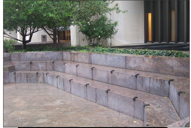
Notches placed to deter skate boarding, in-line skating, etc.
