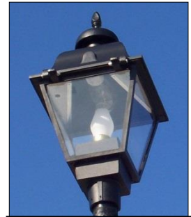
Photo C. The white globe visible to the eye in this post top fixture is decorative; the lamp is in the top of the fixture.
