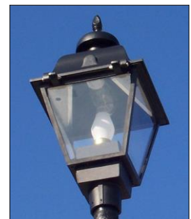
Photo D. The white globe visible to the eye in this post top fixture is decorative; the lamp is in the top of the fixture.
